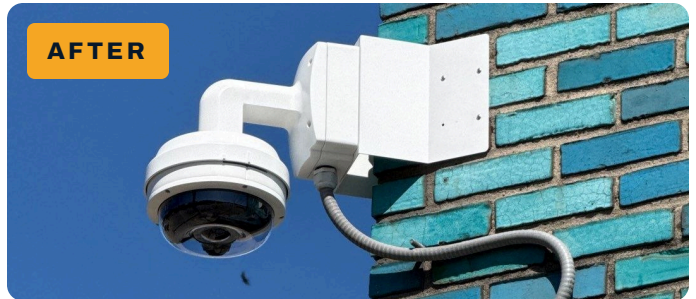
An aging camera and loose cabling replaced with a new high-definition camera and clean, protected wiring.
